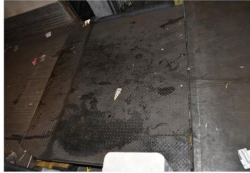
Figure 1. Dock Leveler Lip Extended onto Vehicle Load Bed
